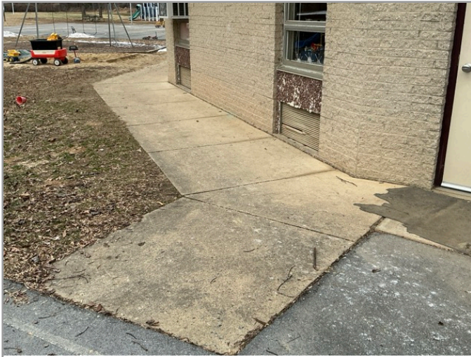
ACCESSIBLE ROUTE TO PLAYGROUND
