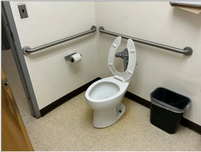
TOILET STALL OVERVIEW
