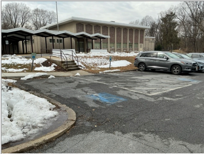
OVERVIEW OF ACCESSIBLE PARKING AREA
